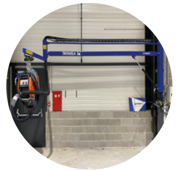
Jib cranes and wire feeder support
